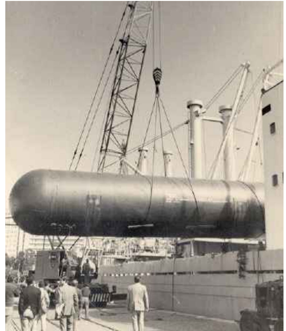
FIRST COMBINED OPERATIONS WITH CRANES AT THE OLD PORT OF BUENOS AIRES
