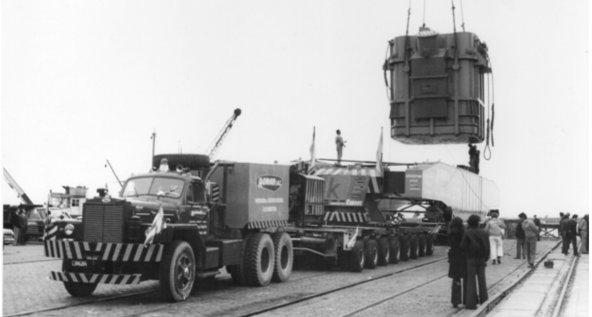
LOADING A 220 TONS TRANSFORMER IN THE PORT OF BUENOS AIRES
