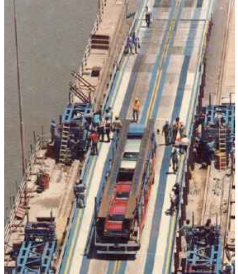
GENERAL MANUEL BELGRANO BRIDGE. ITS REPAIRING, ALLOWING TRAFFIC TO OUR MODULAR OVER BRIDGE
