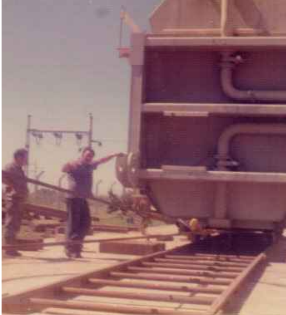
PLACING SIEMENS TRANSFORMERS
