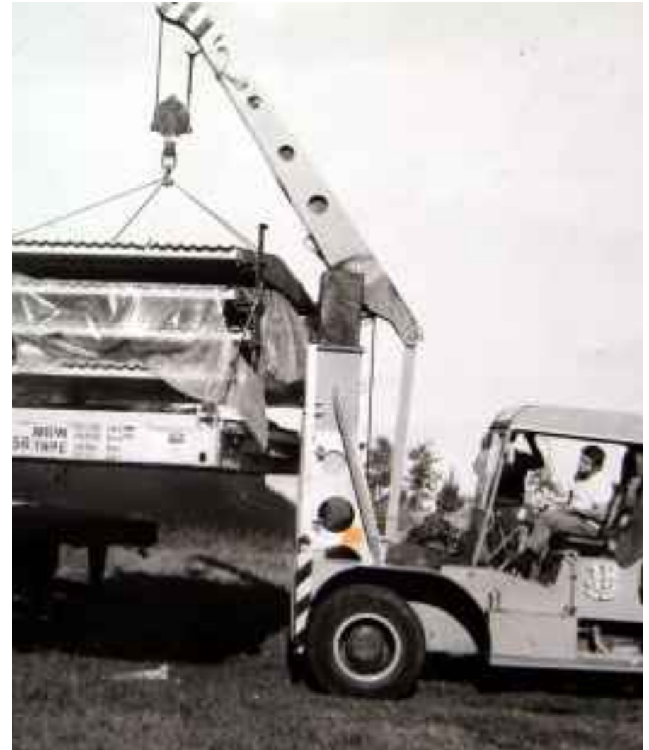
FIRST ROMAN CRANE SAC: TR 22
