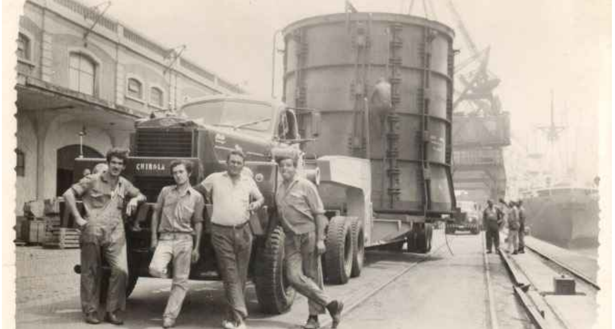
FIRST HEAVY LIFT OPERATIONS IN THE OLD PORT OF BUENOS AIRES
