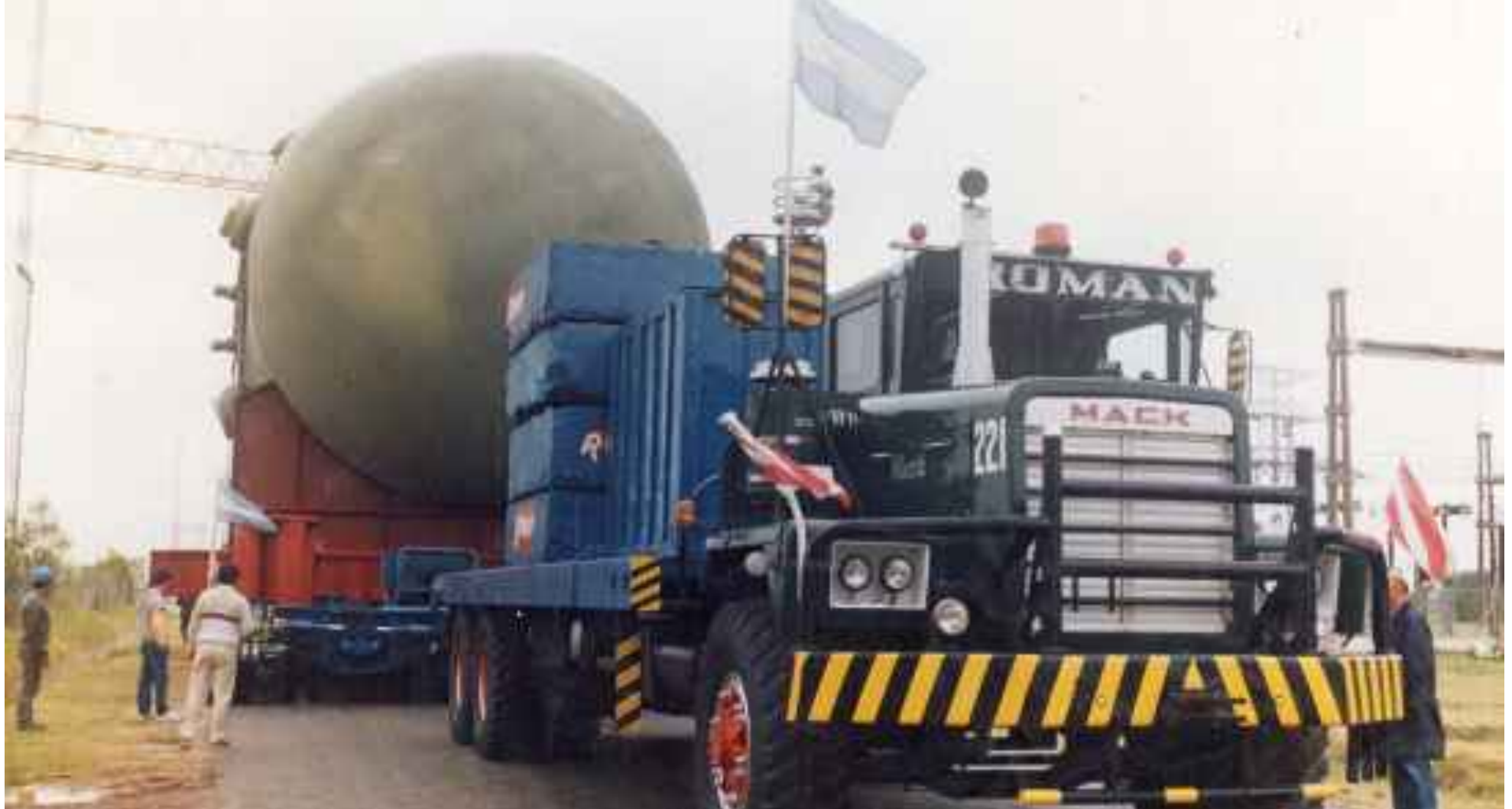
TRANSPORTATION OF THE 870 TONS NUCLEAR REACTOR WITH A MODULAR BOGIE OF 240 WHEELS IN ATUCHA II POWER PLAN - ENACE S.A.
