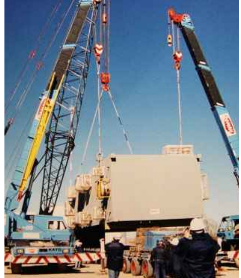
NEUQUÉN-MEGA PROJECT- HOISTING A WATER TREATMENT PLANT
