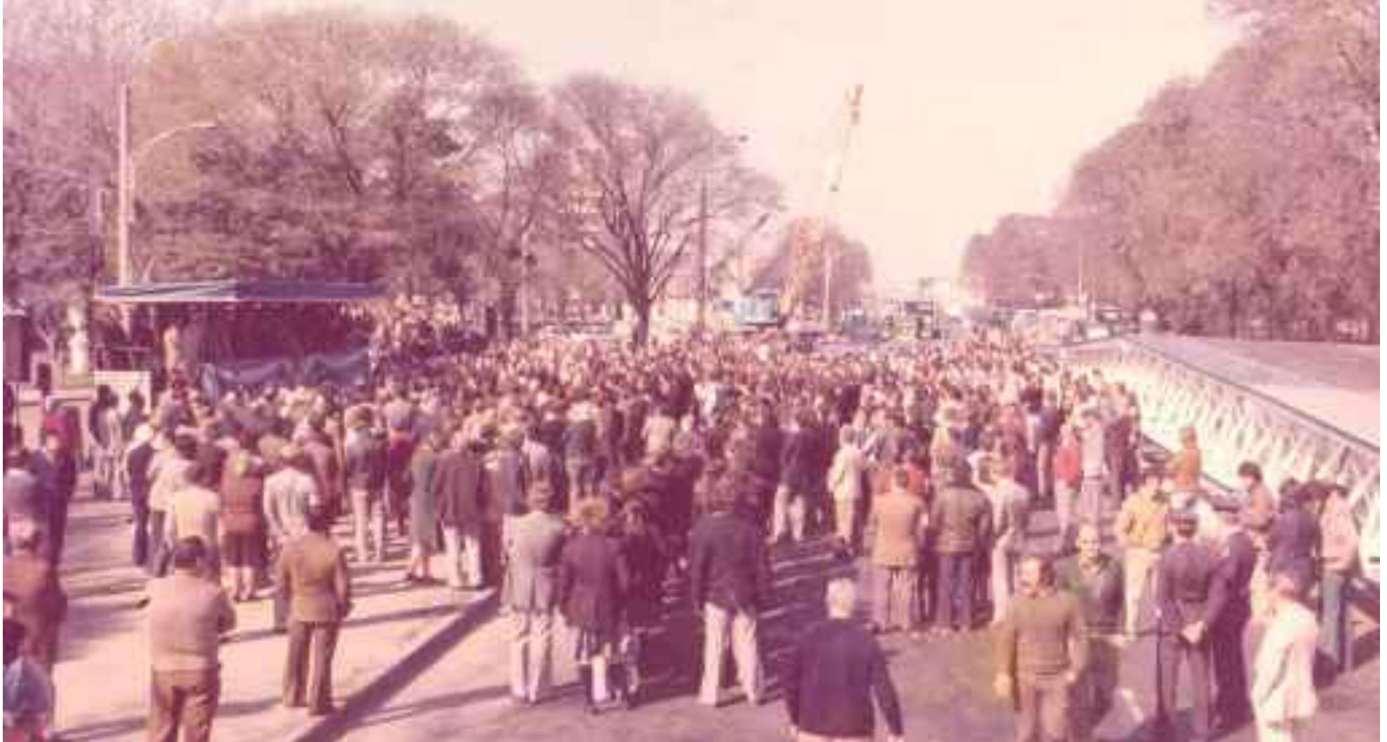
INAUGURATION OF THE OVER BRIDGE ON VELEZ SANSFIELD AV.
