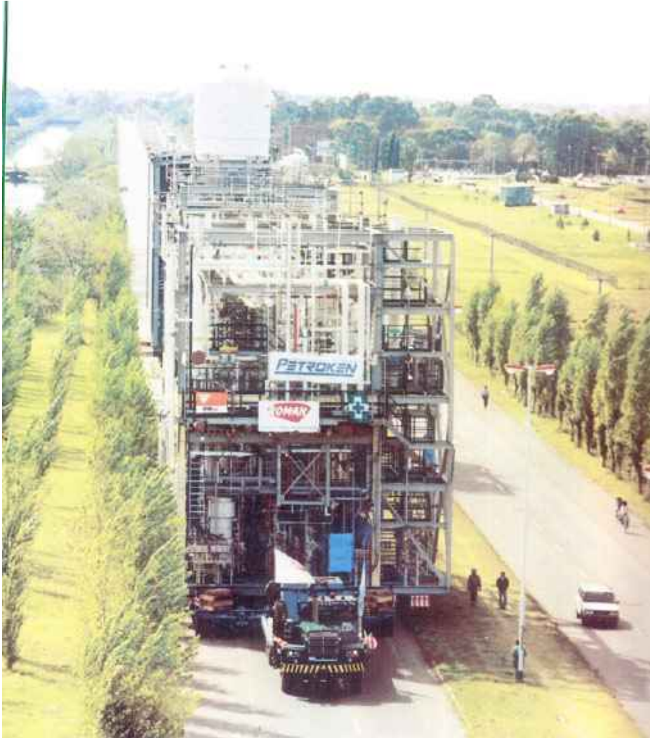
MOVING THE PETROKEN ENSENADA PETROCHEMICAL PLANT
