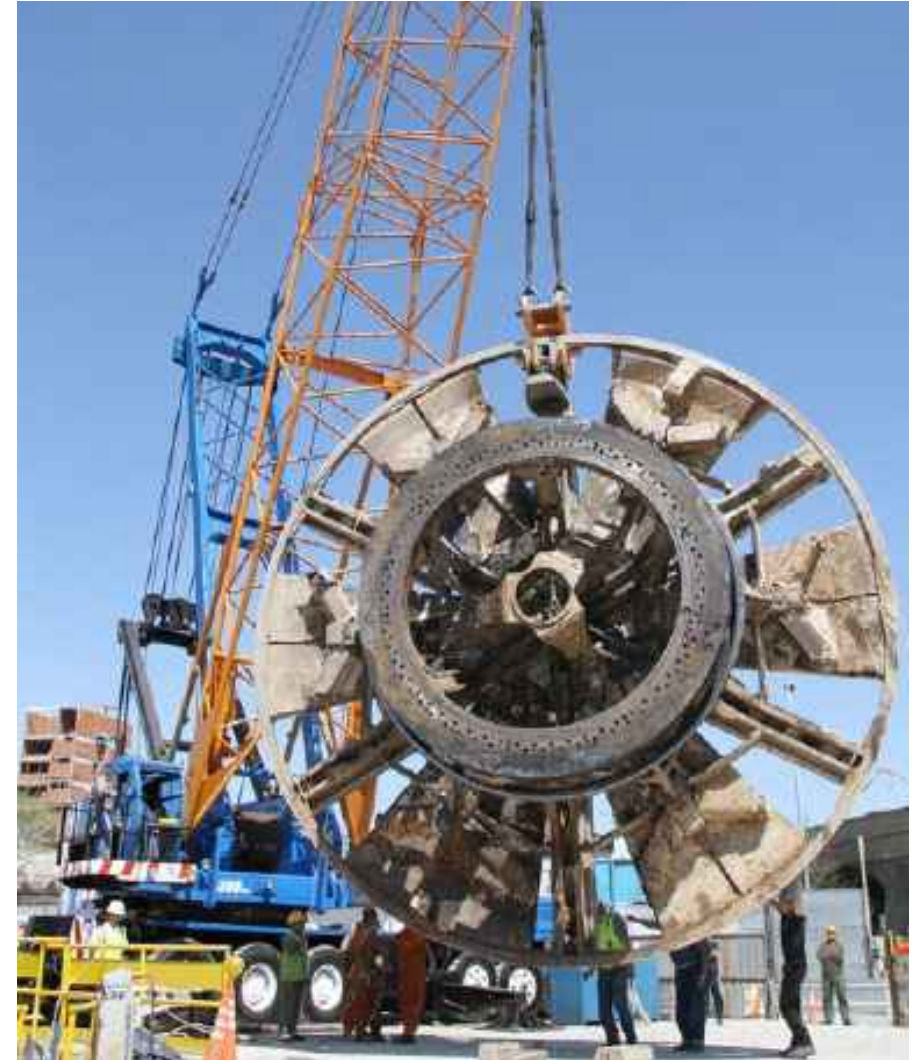
LIFTING AND ASSEMBLING COMPONENT FOR A TUNNELING MACHINE
